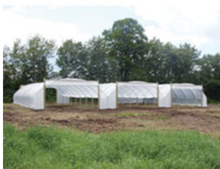
Gutter Connected Field Tunnel
